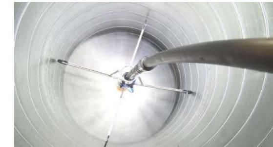
The centering device fixes the brush in the center of the duct.
