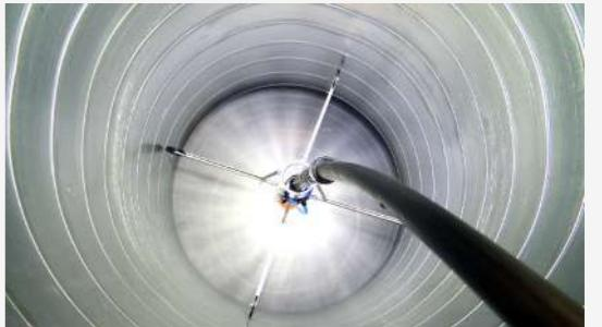
of the duct, avoiding lurches. The wheels allow a better sliding and facilitates the handling of the hose by the operator
